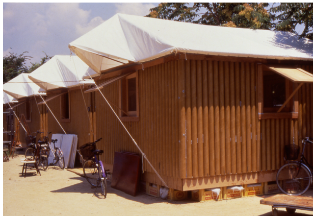
Paper Log House Kobe, Japan, Kobe, 1995 / Photo : © Takanobu Sakuma
