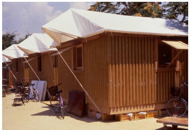
Paper Log House Kobe, Japon, Kobe, 1995 / Photo : © Takanobu Sakuma
