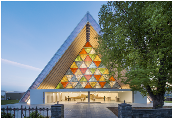
Cardboard Cathedral, Neuseeland, Christchurch, 2013 / Foto : © Stephen Goodenough
