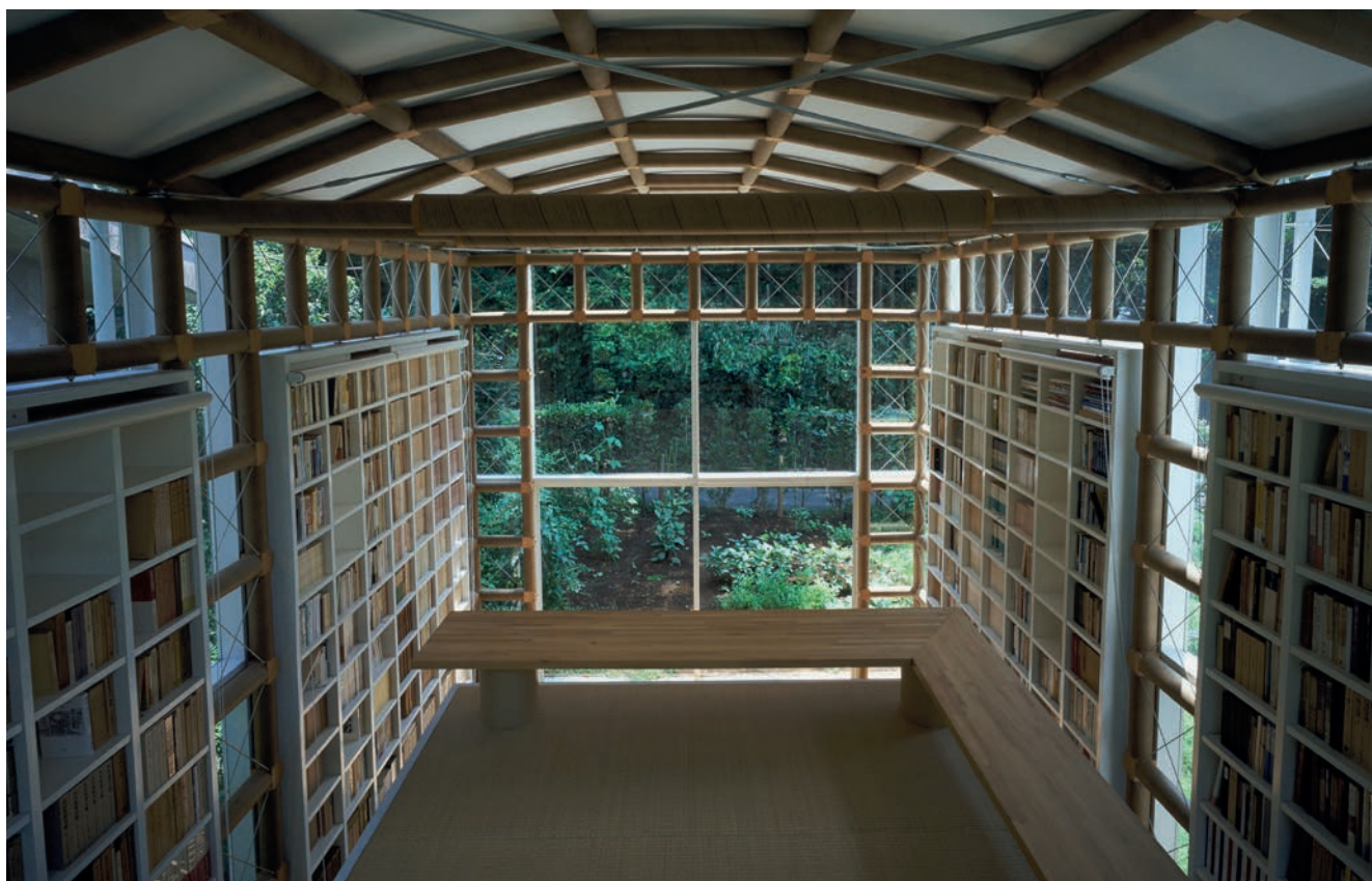
Shigeru Ban, Library of a Poet , Zushi, Japon, 1991 Structure en tubes de papier Photo : © Hiroyuki Hirai
